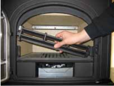
a. Lift and remove the front grate.
