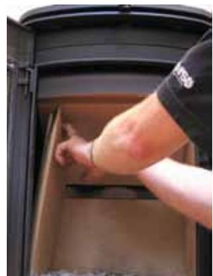
2. Tip the side bricks and remove them from the fire chamber.
