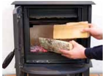
When refuelling your stove, it is recommended that you open the stove door gently for the first 2 - 3 centimetres, then wait for a few seconds for the pressure in the flue to equalise; you are now safe to proceed and open it all the way. By using this technique smoke spillage can be eliminated particularly in poor chimney draft conditions. The stove door should not be opened when the stove is being fired vigorously.
