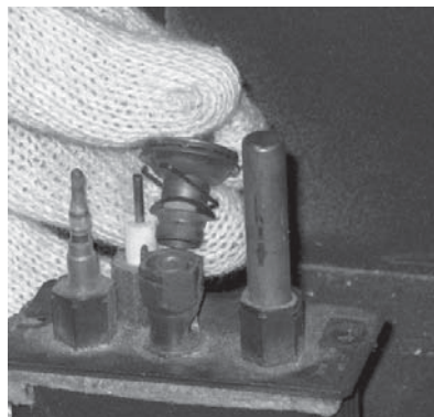
Remove the 2 screws, push Burner Assembly to the left and lift out.
