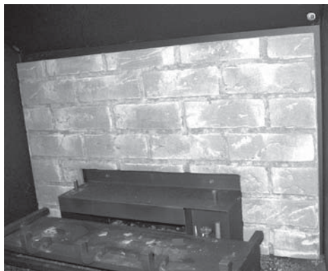
Back Panel Installed
