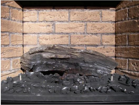
Step 1: Place rear log in notch on left side and on log pin on right side.
